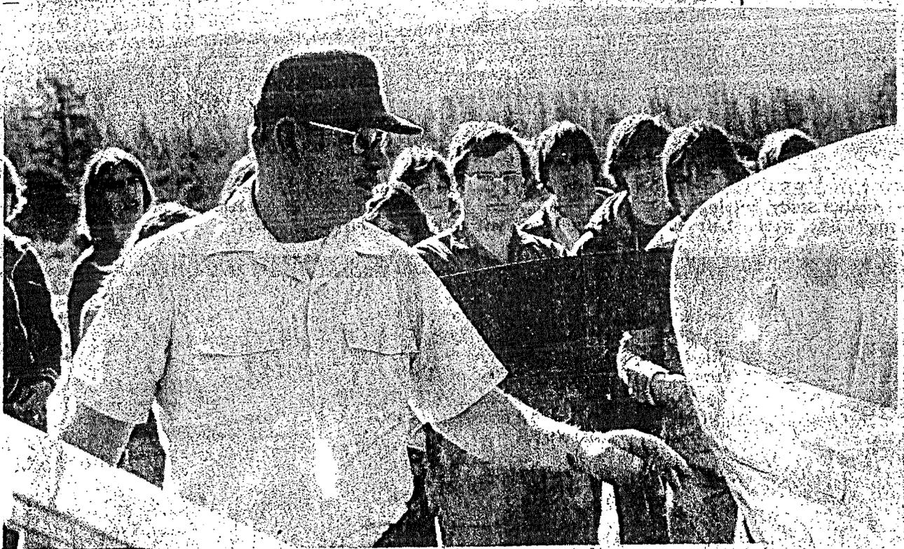
**INSPECTING** the craft before take-off is demonstrated by Jig Taylor, who advises cadets to check the wings and wheels for broken rivets, cracks
