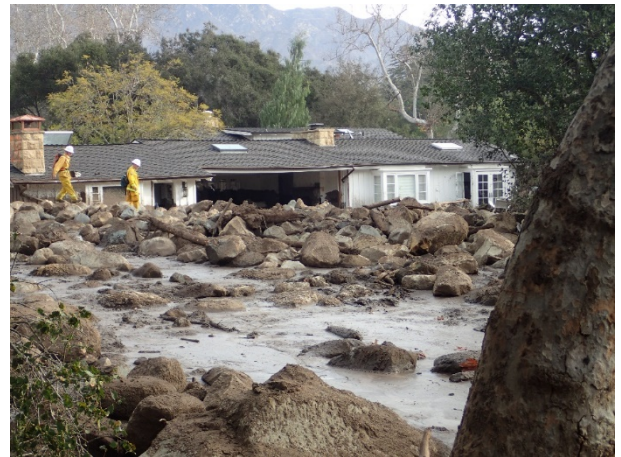
House inundated by Debris Flow – Montecito, 2017 (photo courtesy of USGS)
